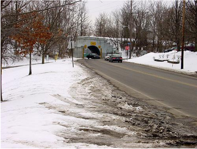
Henry Street Tunnel ca. 2003
