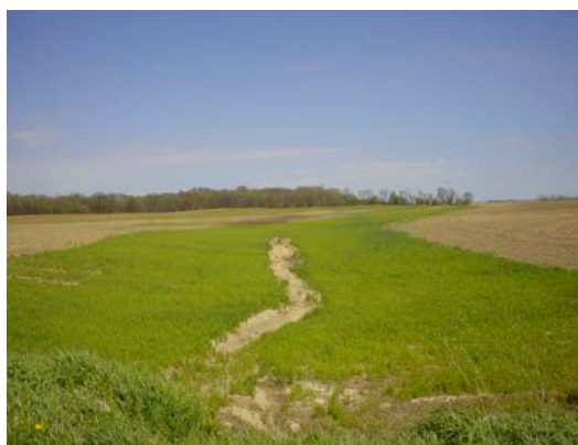
Figure 19: Grassed waterway in need of repair.
