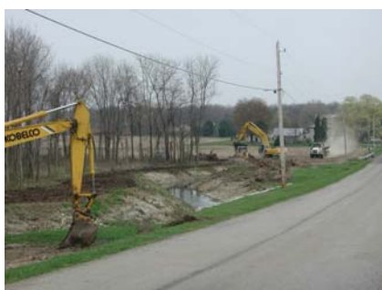
Figure 61: Drainage channel – road culvert maintenance.
