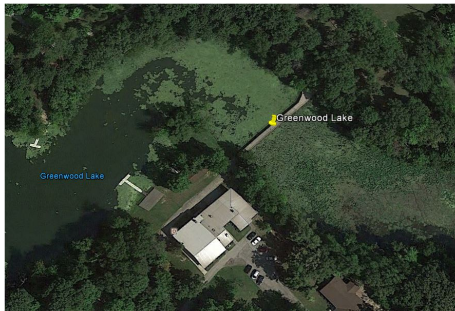
Figure 3: A Google Earth Image of the Greenwood Lake Site
